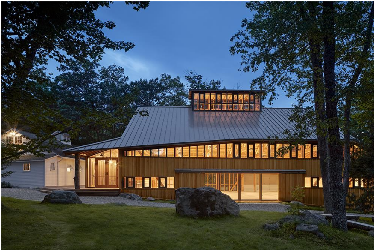
The Perles Family Studio at Jacob's Pillow Dance by Flansburgh Architects. Photography by Robert Benson.
